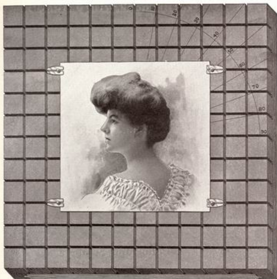
Copy Board in Use—Photograph Held in Place with Four Springs
