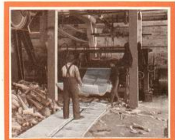
Cutting Veneers for New Departure Bottoms
